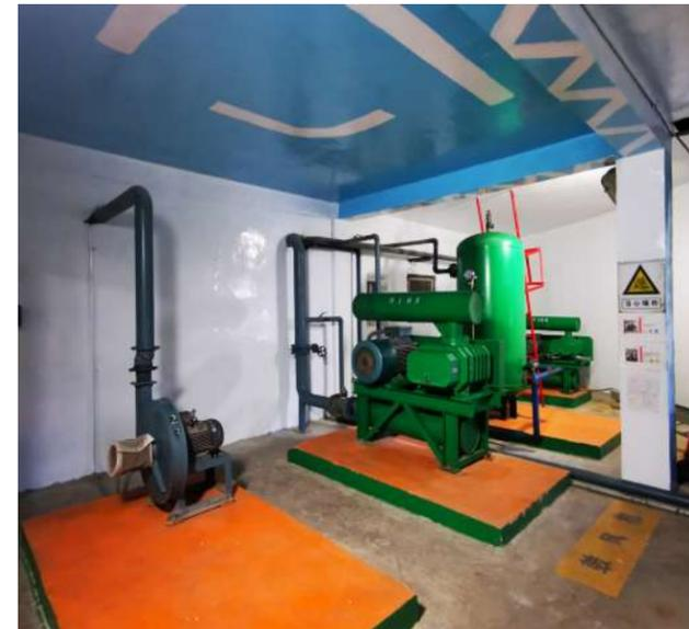
Increase vibration isolation and noise reduction devices for equipment with loud noises
