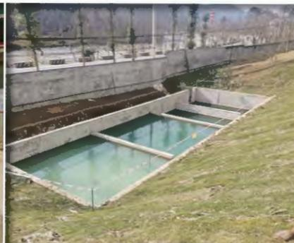
Construct a new three-stage sedimentation pond beside the large silo
