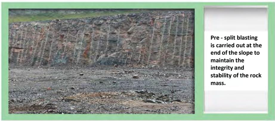
Pre - split blasting is carried out at the end of the slope to maintain the integrity and stability of the rock mass.
